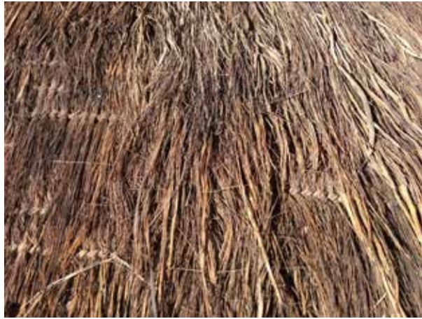
Fig 8. Rendille Mat. Detail of the exterior cladding of a Rendille tent. Note the knotted grid underlying the pile built up by sisal fibers. Photo by Risham Majeed, 2013
