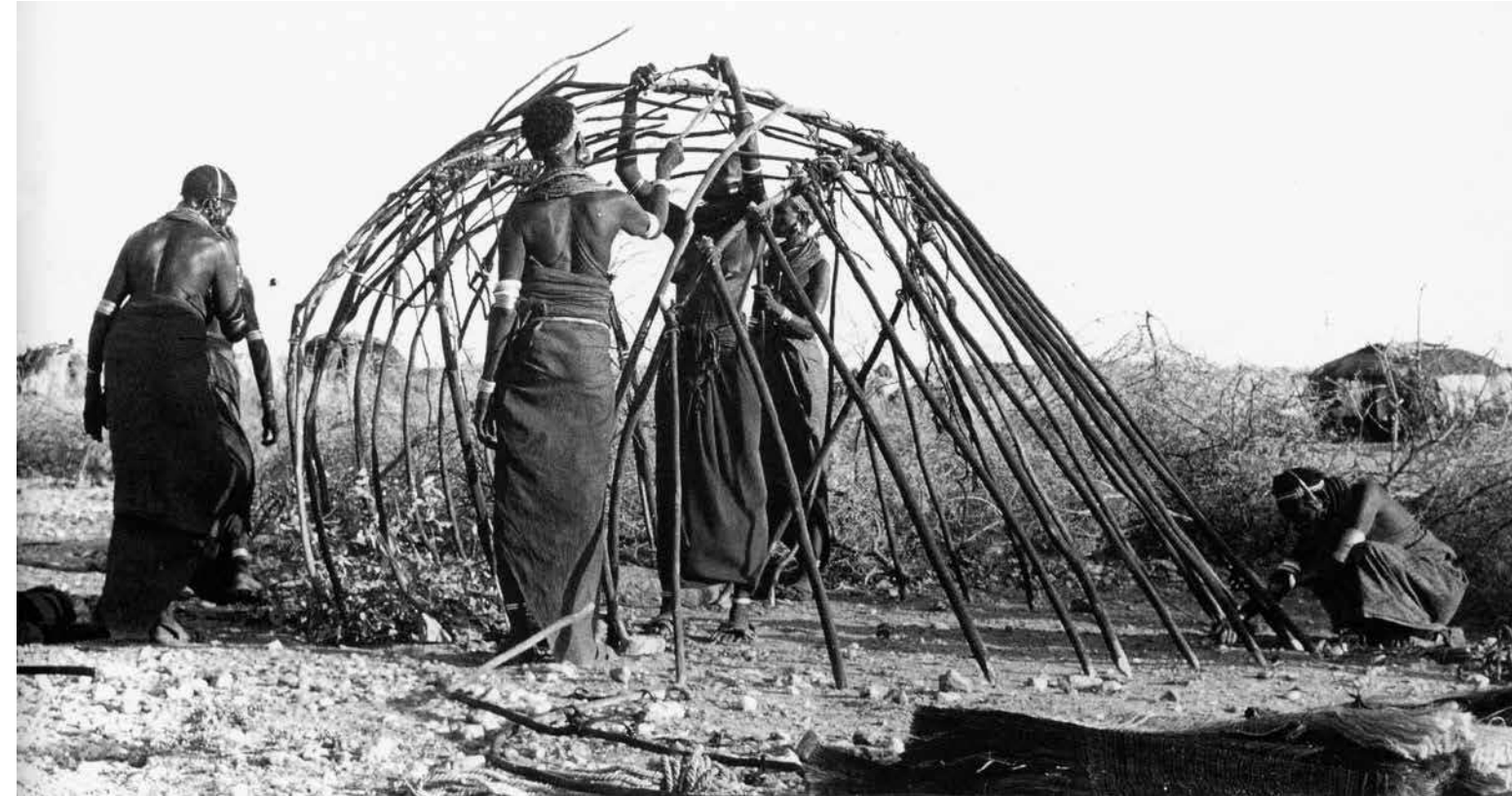
Fig 9. Armature of a Rendille Tent. The frame of the armature in the process of assembly. Note the sturdy straight poles of the lean-to entrance which are not buried but rest directly on the ground. The woman on the bottom right is securing these with rocks. Photo by Anders Grum, Kenya, 1975
