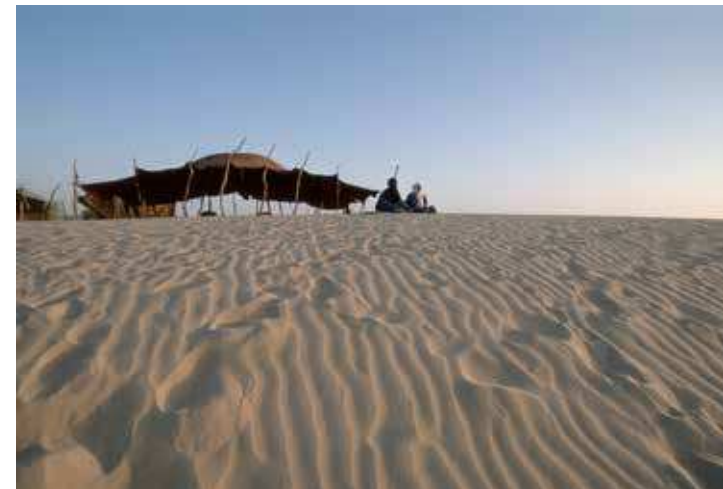
Fig 12. Tuareg Leather Tent, c. 1990s. The tent is open on all sides to allow wind to pass through during the hotter times of the day. The perimeter poles are uncarved acacia saplings that were most likely found on site and not transported from camp to camp. Also note the way the wind leaves patterns like ravines on the desert dunes. Photo by Guenay Ulutuncok
